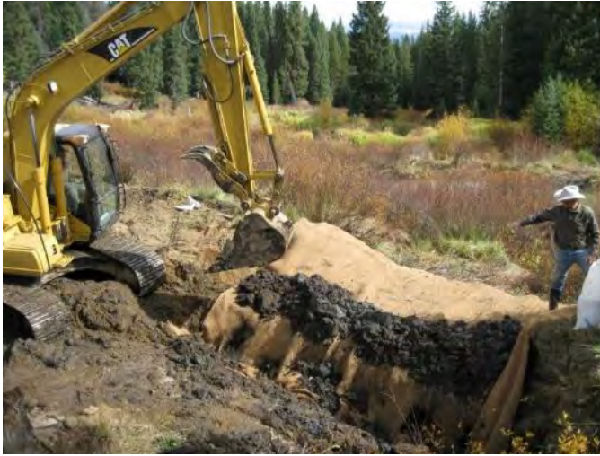
Figure 67: Breached dams were “plugged” with soil lifts wrapped in coir fabric and sod interwoven with live willow stems
