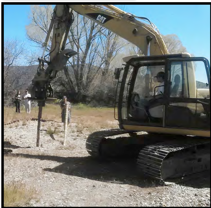
Figure 25: Hydraulic post pounder options. Options include, clockwise, starting from upper left: (a) a hand-held pounder attached to hydraulic power pack, (b) a post pounder attached to bulldozers, (c) a handheld pneumatic post pounder attached to an excavator and (d) a modified excavator with a vibrating pad. Options (a) and (b) take approximately 5 to 10 minutes per post, depending on substrate, and it can be difficult to get to the desired depth. Option (d) takes less than 1 minute per post and can drive posts as deep as needed. All pounders have a metal cylindrical cap that holds the post in place while pounding. Each option has pros and cons to consider, including cost, maximum depth the posts can be pounded, substrate type, operator strength and expertise, and the amount of likely riparian and instream disturbance. Photo credits: (a) Nick Weber, Ecological Research, (b) Mark Cookson, USFWS, (c) Peter Thamer, Siskiyou County Resource Conservation District, and (d) Julie Ashmore, Okanogan Highlands Alliance.
