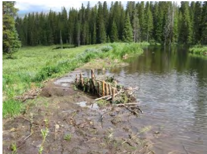
Figure 68: A PLWW was constructed on one repaired dam to temporarily fortify a nick point while we were waiting for beaver to reoccupy the site
