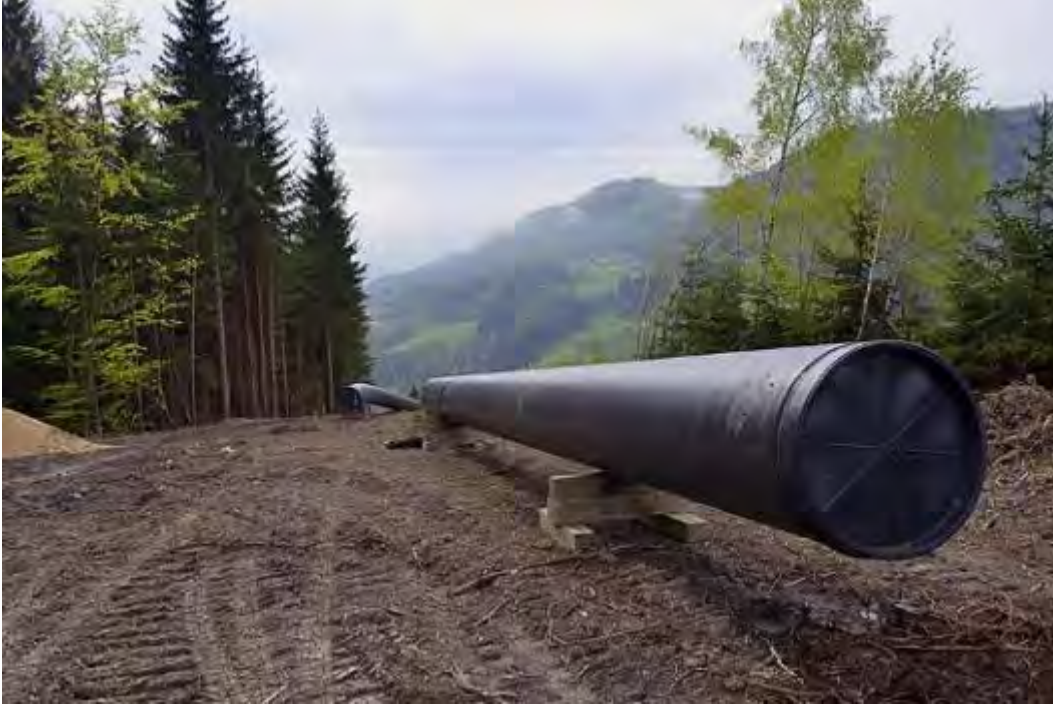
Figure 46. Pipeline development showing size of pipe and common width of clearing.
