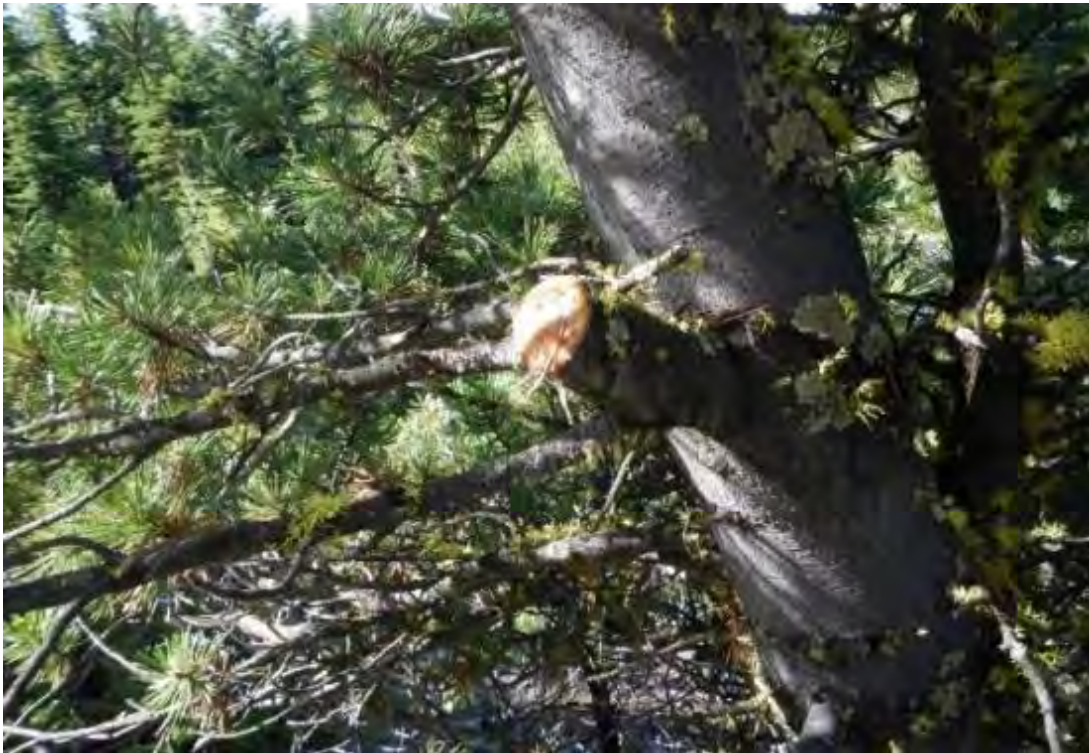
Figure 50. Branch stub left after improper pruning to widen trail access; branch should have been cut to stem.
