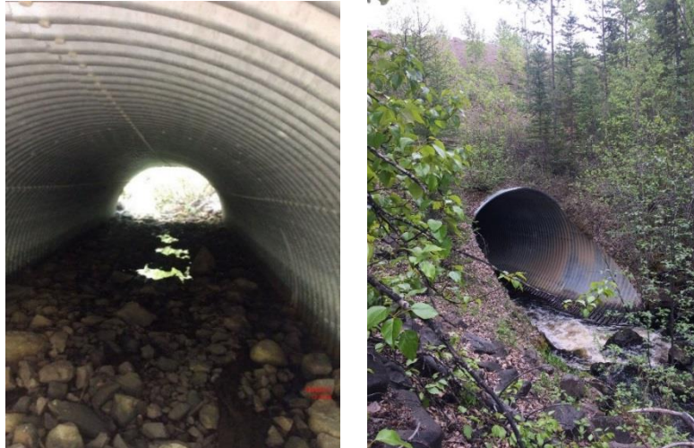
Figure 12 Crossing 1216: Arch Culvert Situated Upstream of Possible Fish Barriers (Right). Crossing 285: Closed Bottom Structure (Left).
